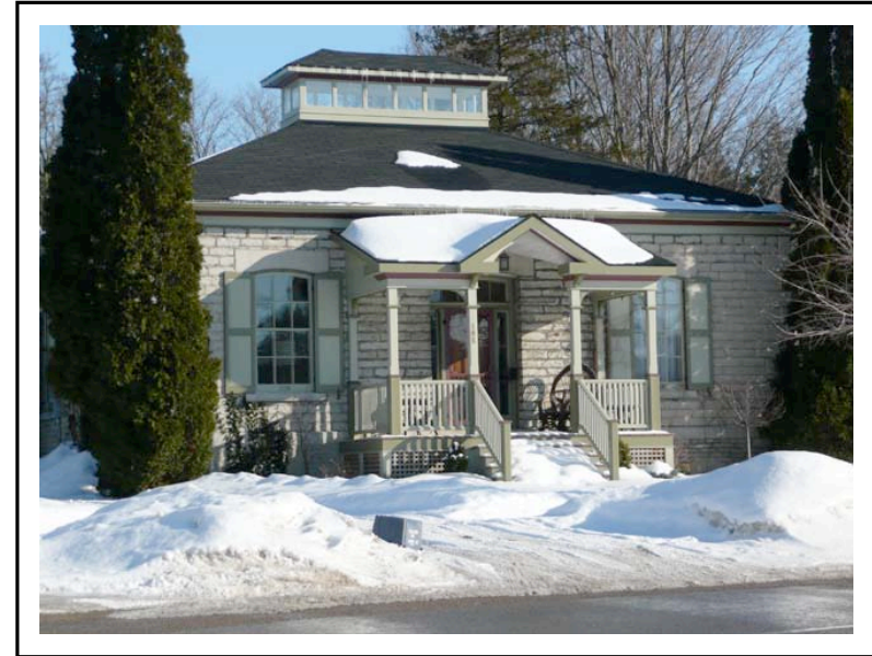
Alterations to porch designed to be compatible with existing house in scale, details and colour (note: property not in District, but shown here for illustrative purposes)
