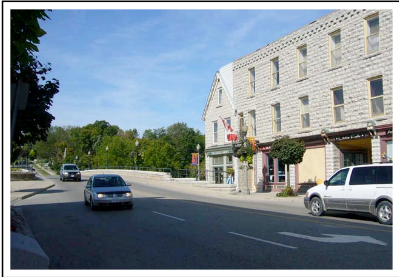
Prevalent use of locally quarried limestone as a building material
