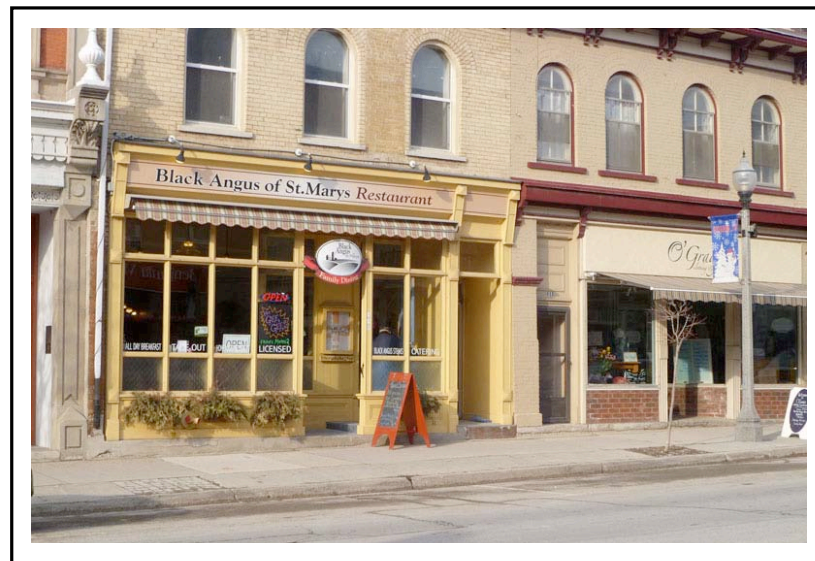
Traditional storefront restored with retractable awning and appropriate use of signboard
