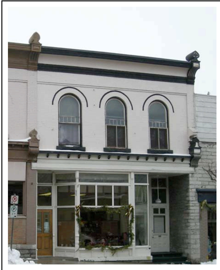
Recessed entrances in original storefronts should be retained
