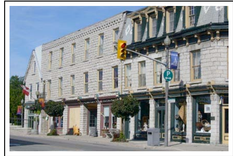
Limestone exteriors are predominant, Queen Street West
