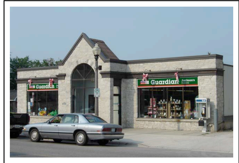
Complementary new building in District—masonry façade in neutral palette with cornice banding and decorative stone surrounding arched front window (credit: St. Marys Heritage Committee)
