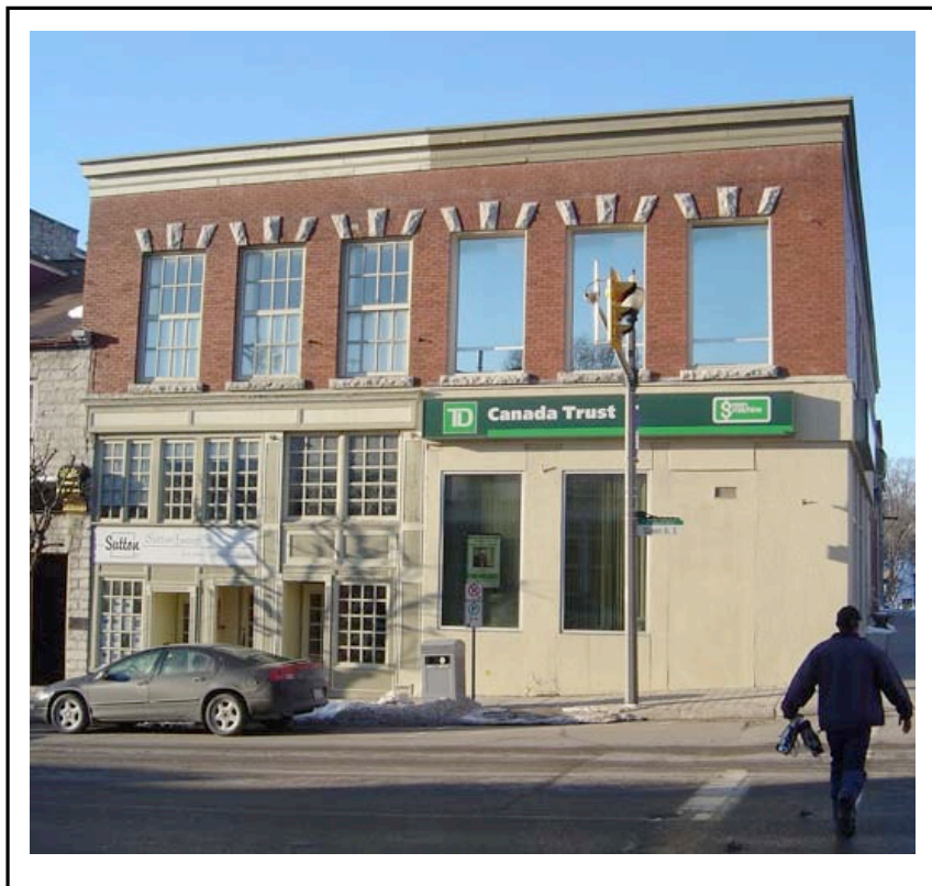
Storefronts should be designed as an ensemble—avoid carrying the distinction between tenants above street level (credit: St. Marys Heritage Committee)
